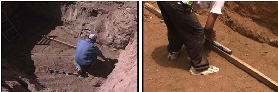
Figure 4. Leveling the bottom of the tank hole.
