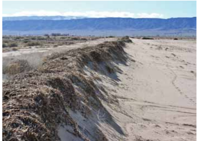
Figure 6: Berms are semi-permanent features on the landscape that provide effective reduction of blowing sand. (Prevailing wind blows from right to left.)
