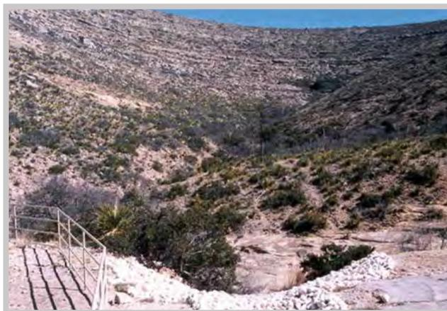
*Drainage from the pavement had caused erosion and sedimentation problems until armored drainage ditches were constructed. Also, unrestricted trail erosion was brought under control using pipe fencing, as seen on the left.*
