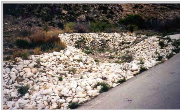
*Sediment Basin – an armored basin was constructed to capture stormwater runoff from the paved areas and prevent erosion and sedimentation.*
