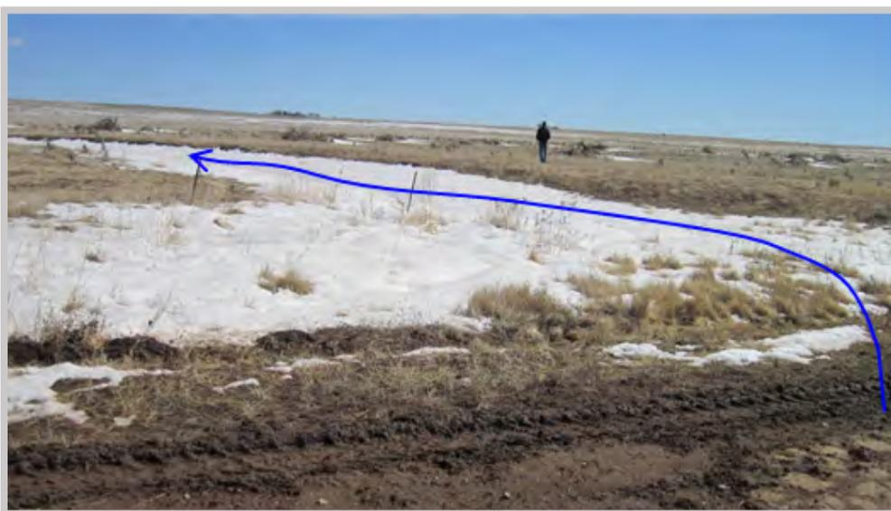
*Road runoff and sediment entered the playa through a ditch running from a low water crossing straight to the playa.*
