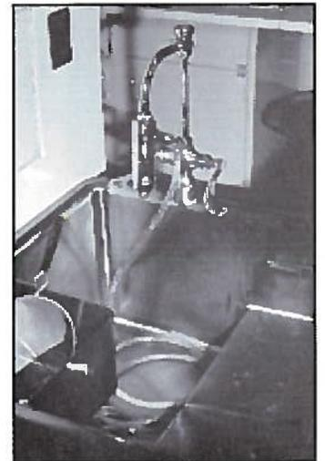
Figure 16 shows the generally accepted installation requirements—note that no shutoff valve is downstream of the device that would otherwise keep the atmospheric vacuum breaker under constant pressure.
