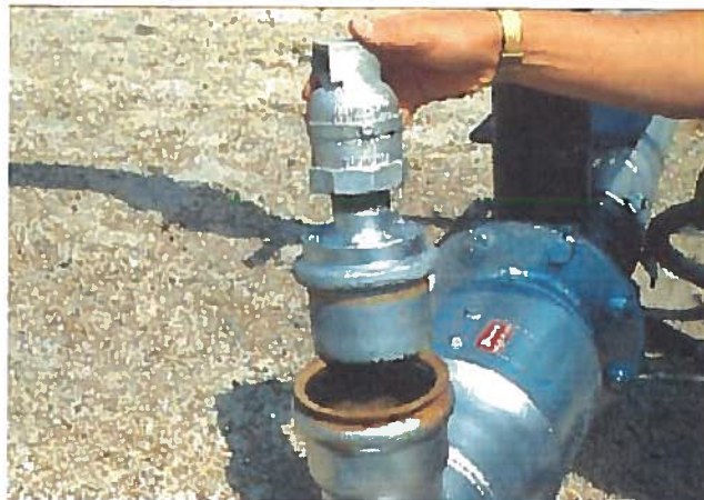
Four inch diameter inspection port allows you to see if the check valve is working when the water pump is off. Below the 4 inch opening you can also see the low pressure drain.
