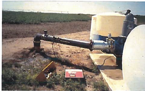
How the chemigation check valve and other connections protect the water supply (well).
